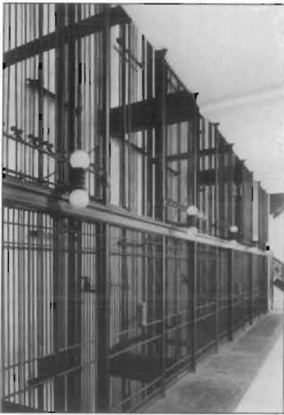
Both function and design elegance are evident in this row of cast iron elevator cages and light fixtures adorning an early-20th century commercial building.
