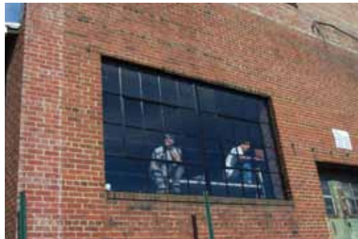
Recommended: [33-35] Original metal windows were appropriately repaired as part of the rehabilitation of this historic industrial building.
