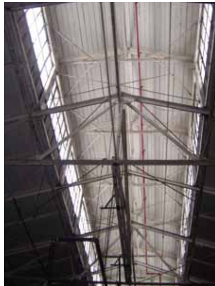
[12-14] Roof monitors provide natural light in historic industrial buildings
