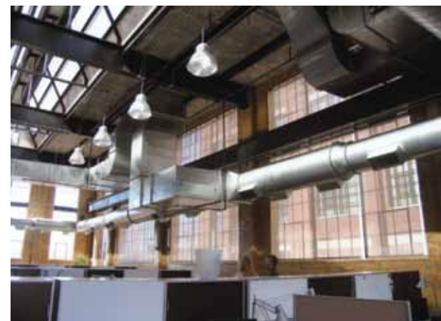
[5-6] Large windows and a roof monitor provide natural illumination in a historic industrial building.
