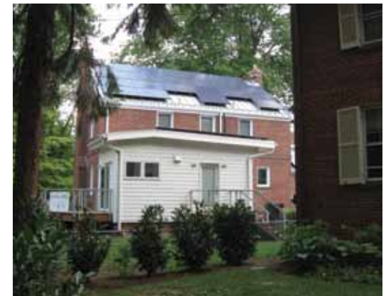
Not Recommended: [75] Solar roof panels have been installed at the rear, but because the house is situated on a corner, they are highly visible and negatively impact the character of the historic property.
