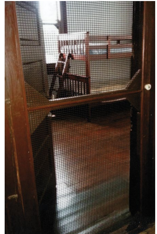
[31] An interior screen door at the entrance to individual apartments is a historic feature traditionally used to help circulate air throughout the building.
