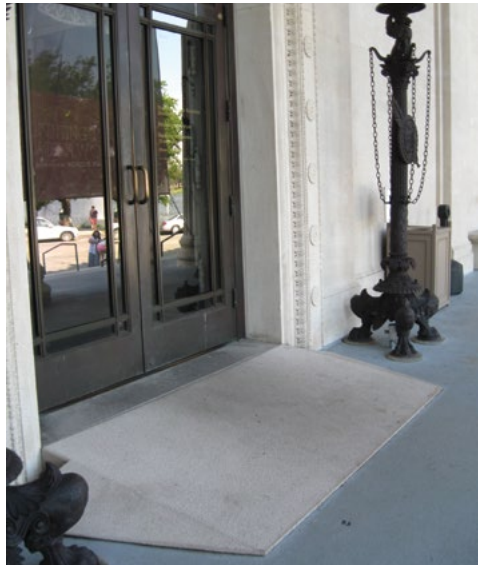
[26] A temporary ramp—unobtrusive and easily removed—facilitates access to the entrance of this museum and does not affect its historic character.
